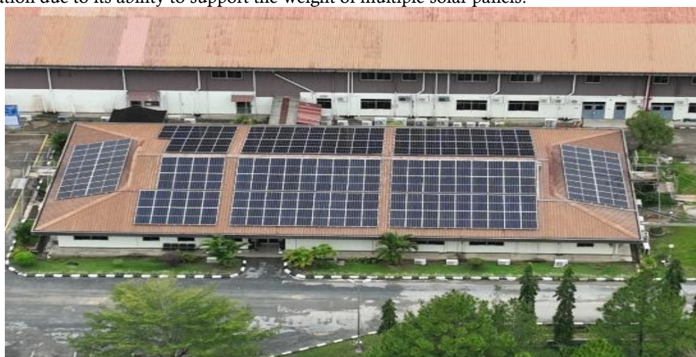
Figure 2. PV Module Placement on the Roof of the Administration Building
