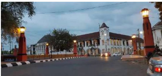
Figure 13. Berok Bridge (Source: Author's Document, June 2019)
