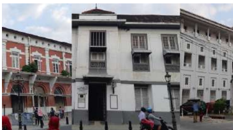
Figure 9. Fenestration Façade on the South Side. (Source: Author's Document, June 2019)
