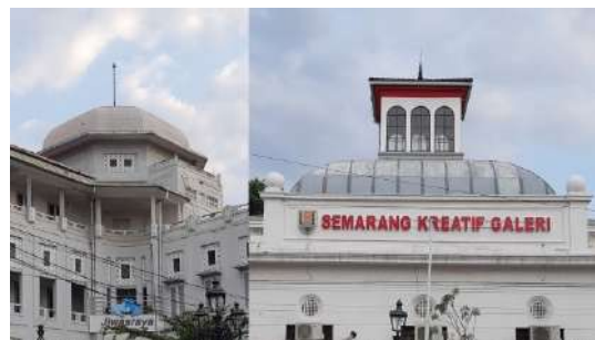
Figure 11. Roof and Tower on the South Side Buildings (Source: Author's Document, June 2019)
