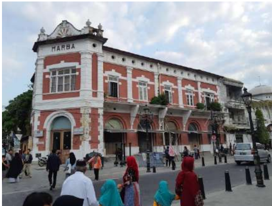
Figure 29. Table Building Lighting (Source: Author's Document, August 2019)
