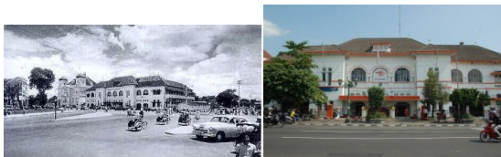
Figure 2. Main Post Office Building Source: https://kebudayaan.kemdikbud.go.id/ (accessed on January 29, 2020)
