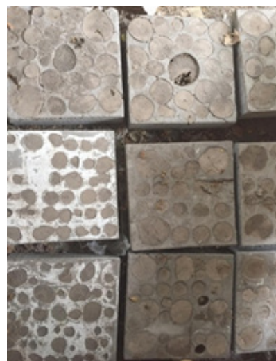
Figure 2. Installation of wooden concrete floor blocks after 5 months
