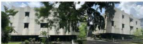
Figure 4. Building Library L7, View from North (left hand photo); 3D View (right hand photo) Source image: Author, 2021
