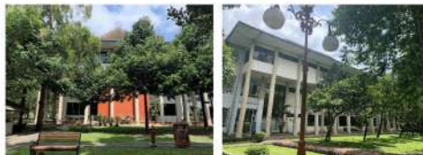
Figure 5. Building Library L6 View from East (Left hand photo); View from South (Right hand photo) Source image: Author, 2021
