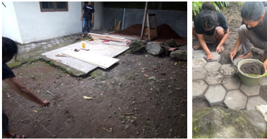
Figure 3. Site Preparation Source: Author
