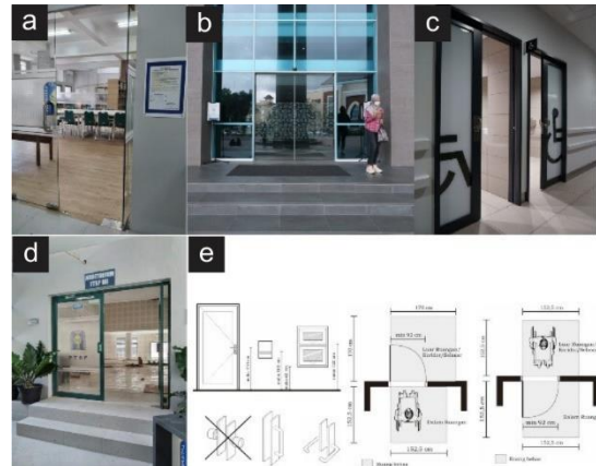
Figure 7. Accessible Door, a) Gen 2, b) Gen 4, c) Gen 4, d) Gen 2, e) Accessible Door standard Source: Author, 2024
