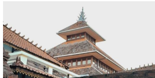
Figure 16. The Three-tiered Roofs of Menara Kudus Mosque Source: Author, 2023
