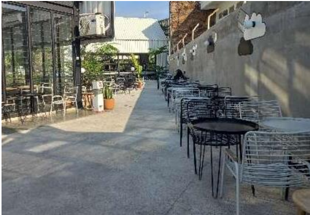
Figure 16. Unfinished Floor Concrete
