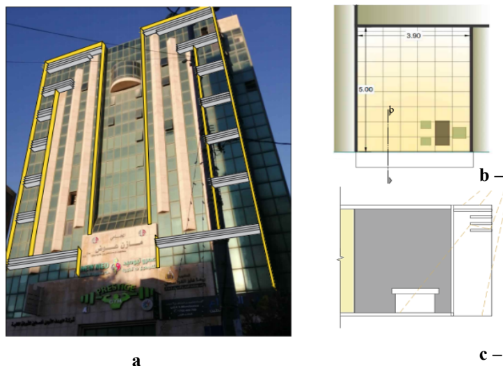
Figure 12. a– The proposed shading devices for the South-oriented Golden tower, in which the shading system covered most of the glazed façade and affected the transparent appearance. b– A plan illustration of the added shading consists of side fins, 1m overhang, and 1 m louvre. c– section b-b of the added shading
