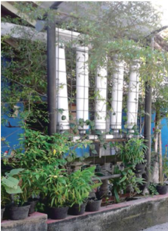
Figure 3. Shelter of plants and rainwater saver in Proklam Sekip Kadipiro Surakarta (Source: Presentation from Kampung iklim Sekip Kadipiro, 2015)
