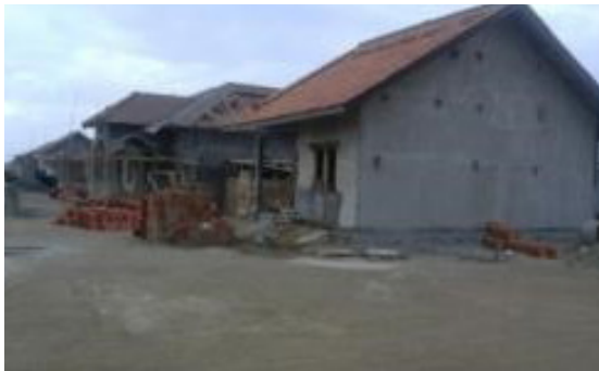
Figure 6. Relocation of affected residents in Kulonprogo under construction
